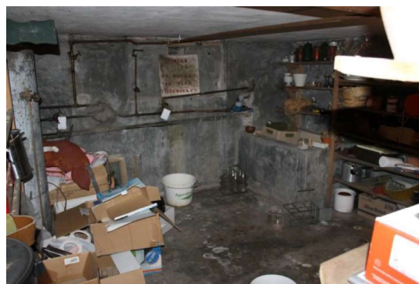
Pekelbak in kelder
