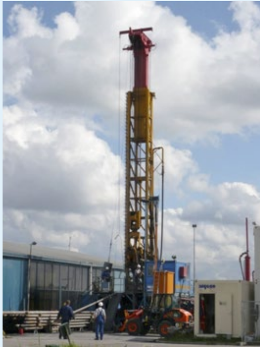
Geothermieboring in Bleiswijk (bron: http://www.geothermie.nl/index.php?id=23; )
