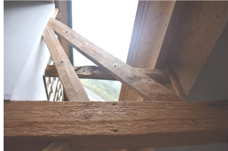
Houten spant op verdieping linker woning.
