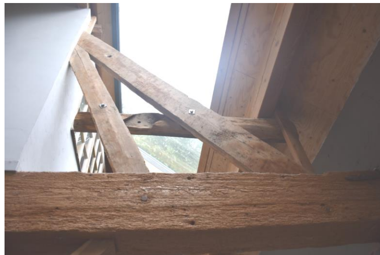
Houten spant op verdieping linker woning.
