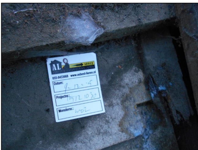
Foto 11: Woning 1: Dakbeschoot (M02AA)
