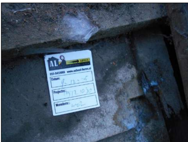
Foto 11: Woning 1: Dakbeschoot (M02AA)
