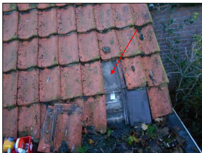
Foto 12: Woning 1: Dakbeschoot (M02AA)
