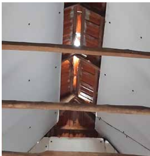
Opening in dak.
