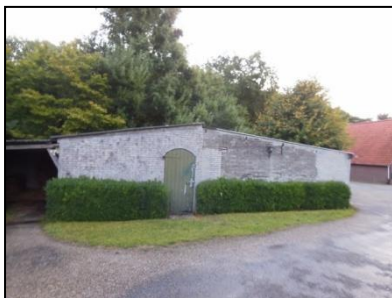
Figuur 3. Te slopen berging.
