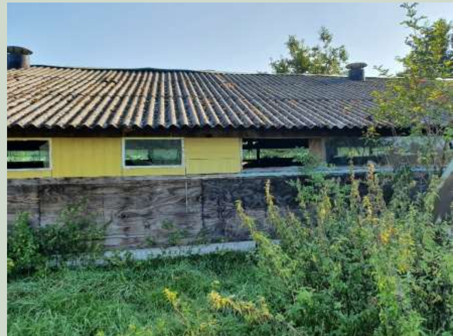
Te slopen stal
