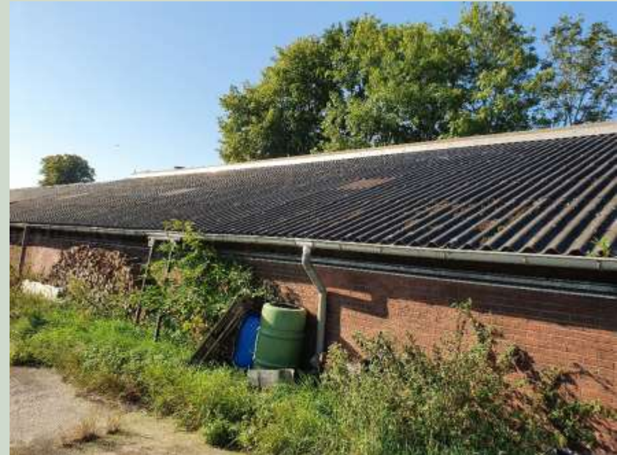
Te slopen stal
