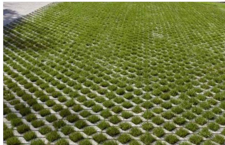
Referentie, half open bestrating parkeren, grasbetonstenen
