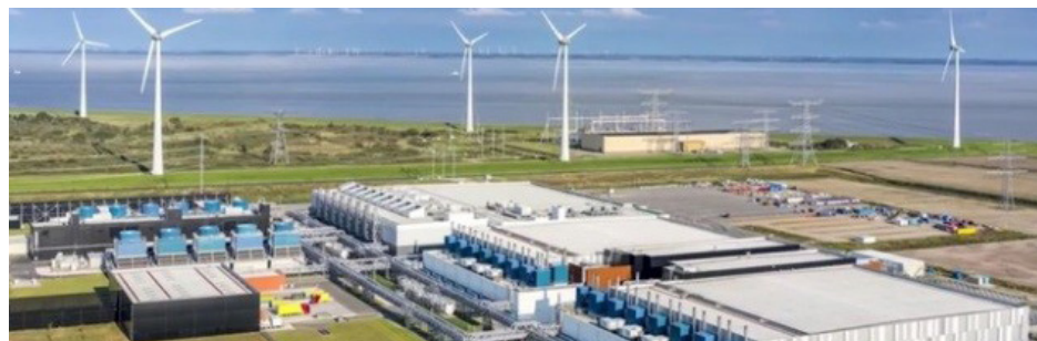
Google datacenter Eemshaven
