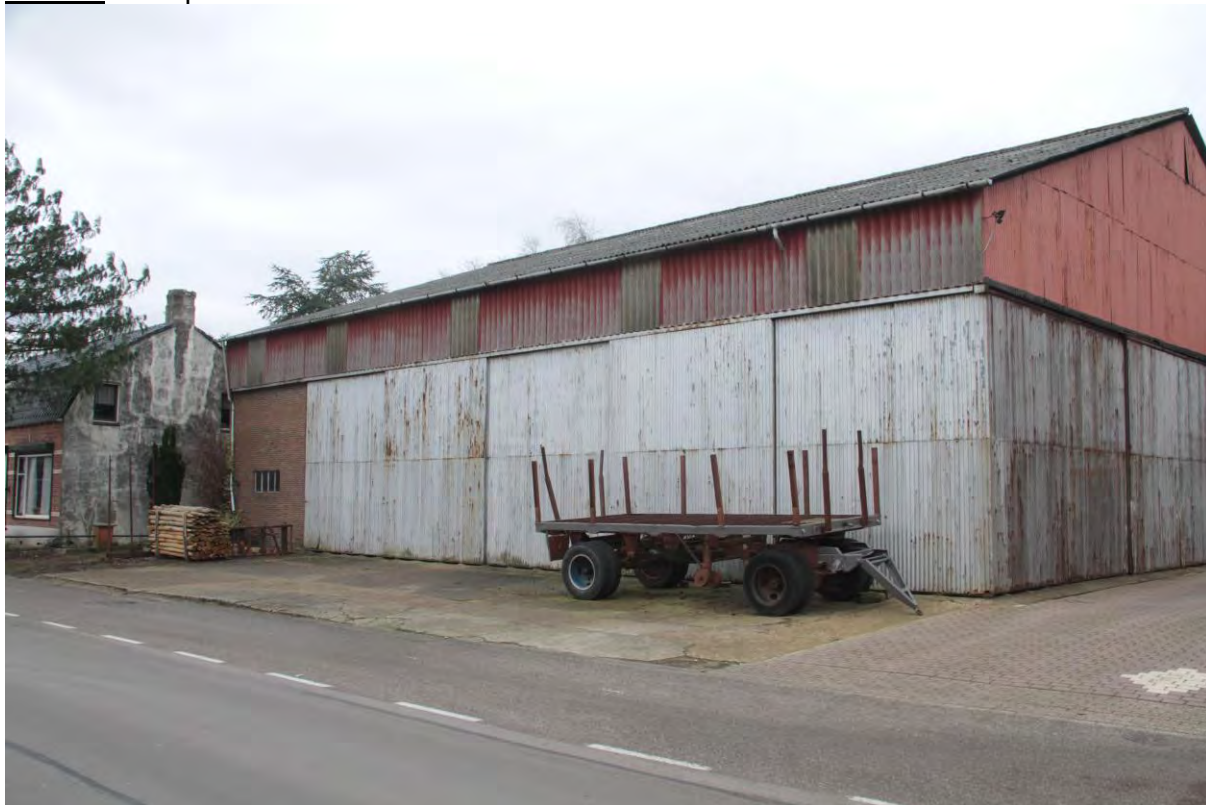
Foto 1. Te slopen loods.
