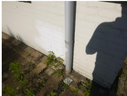
Pvc hemelwaterafvoer
