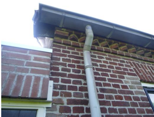
Pvc hemelwaterafvoer
