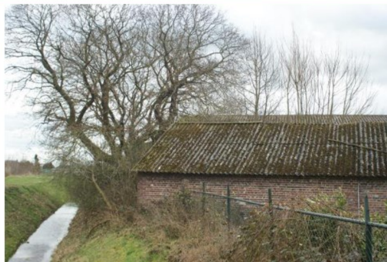
18 Talud langs sloot
