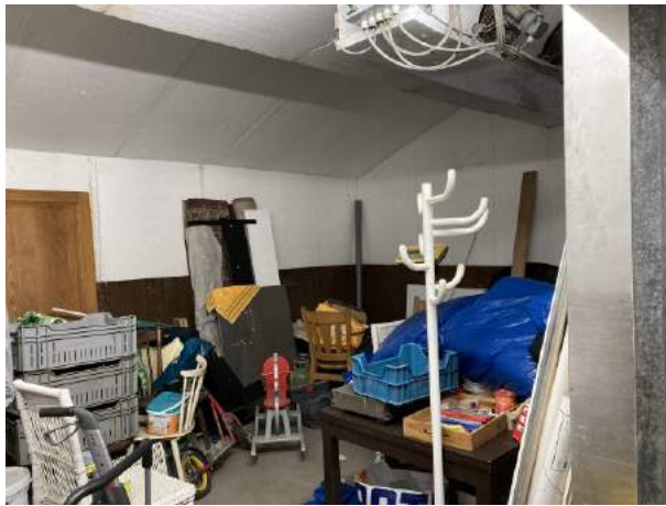
Foto 7 Koelcel in loods
