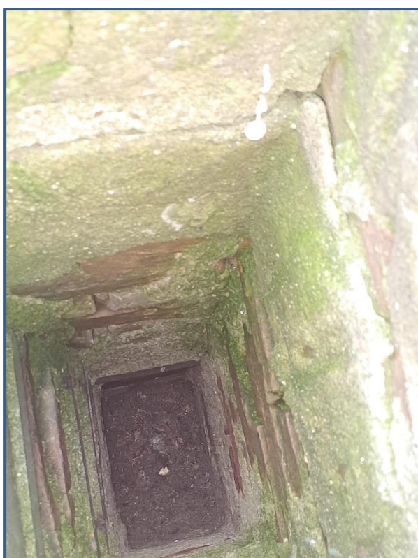
Opening schoorsteen plat dak
