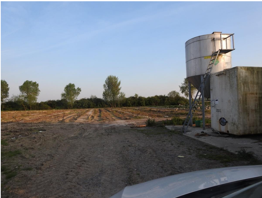
Foto 3. Te slopen silo's
