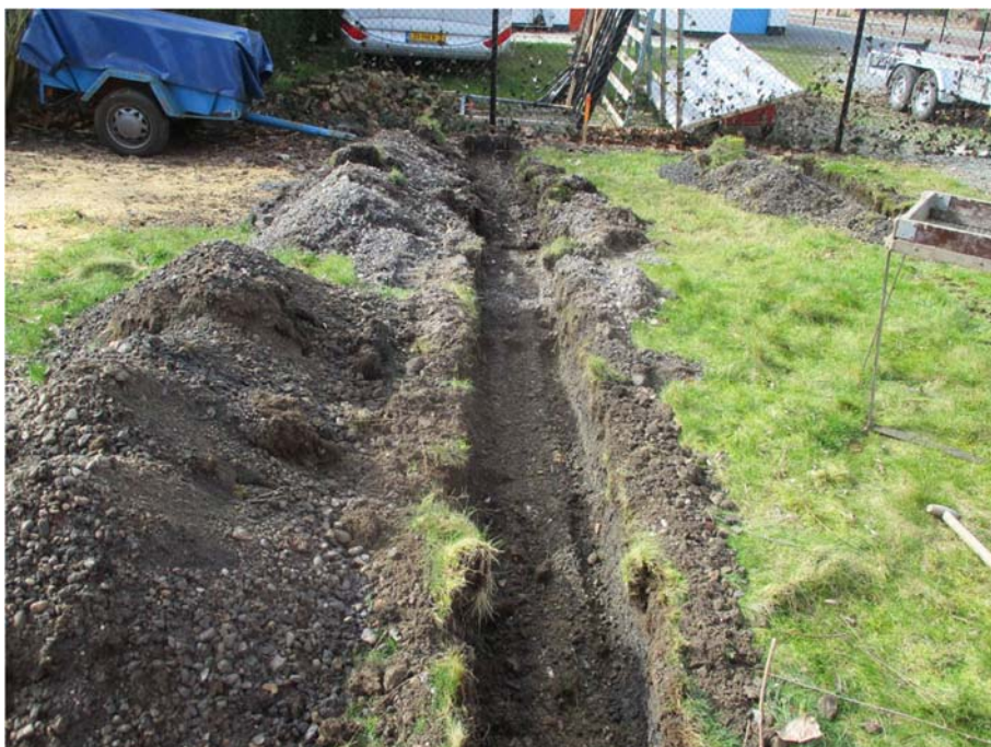
IMG_0208. Sleuf SL01A. Sleuf SL01B rechts.
