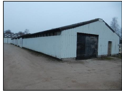
Figuur 11. Te slopen loods.
