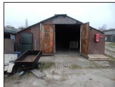
Figuur 8. Te slopen loods.
