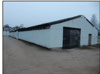
Figuur 11. Te slopen loods.
