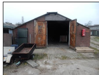
Figuur 8. Te slopen loods.
