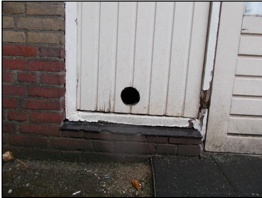
Foto 3. Opening in bebouwing.
