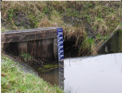
Stuw, peil 1490 (10 cm water over de stuw)
