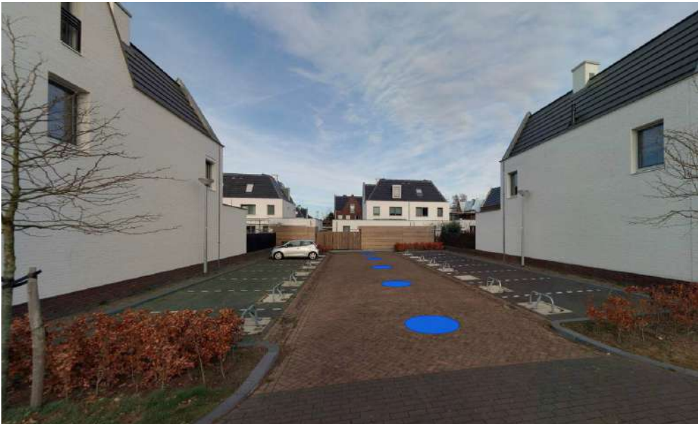
Parkeren in parkeercoffer
