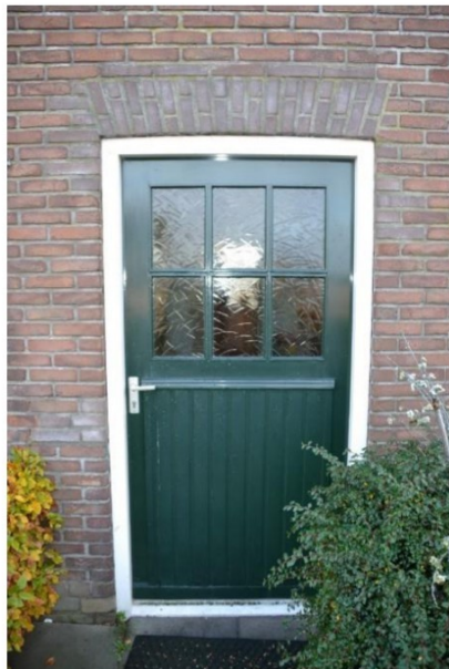
Later aangebrachte deur in de vm. stal.
